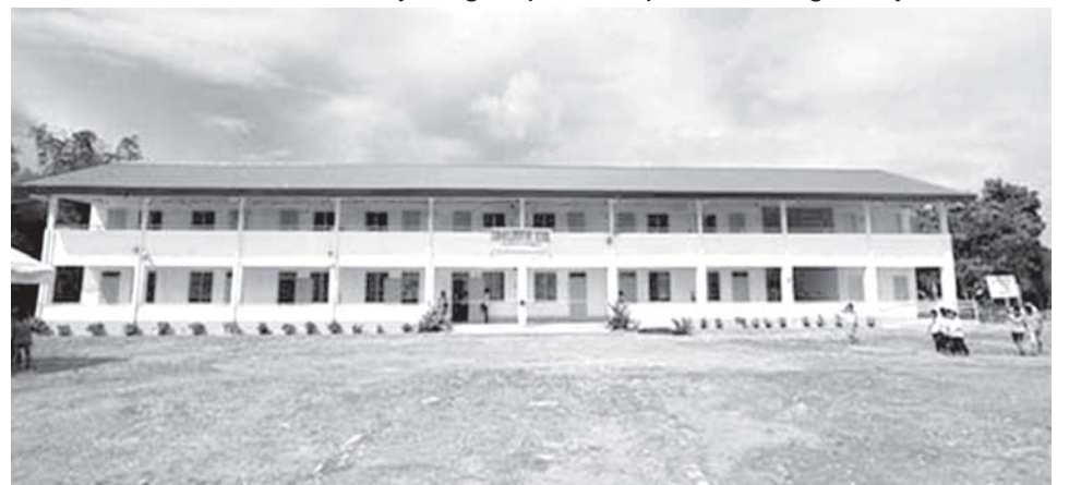
The new two-storey, eight-classroom building of Cano-an Elementary School in Estancia, Iloilo can withstand winds up to 250kph.
